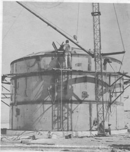
RADAR SITE WATER TOWER NEARS COMPLETION
